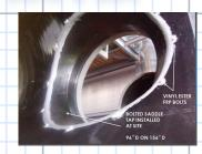
Once the system is operational, using the **ATS HotTap™** procedure, taps can be added to the live systems without pressure loss.
